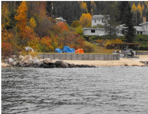
Retaining walls and stone groynes (Segment 68)
