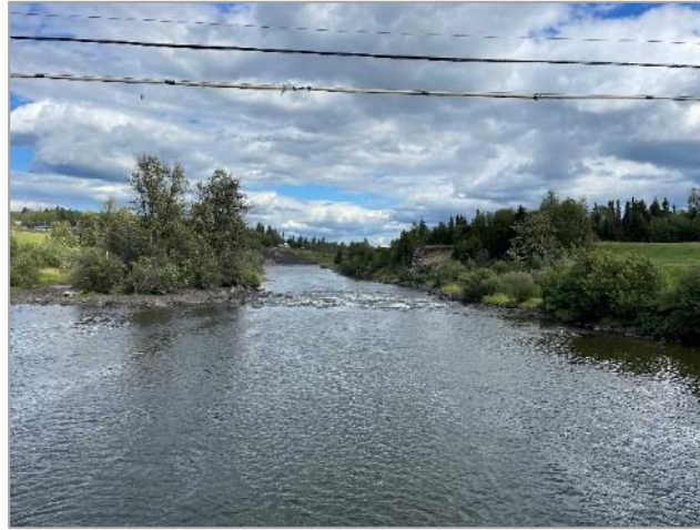
Photo 1. Hydrologic control structure downstream of bridge on Nautley River. Photo taken from bridge (Segment 35).
