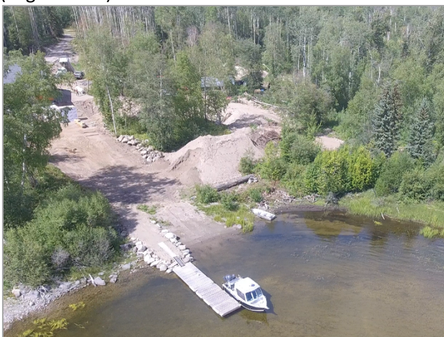
Photo 35. Example of recent development at/below high water mark (Segment 12). Note large pile of soil in close proximity to edge of water.
