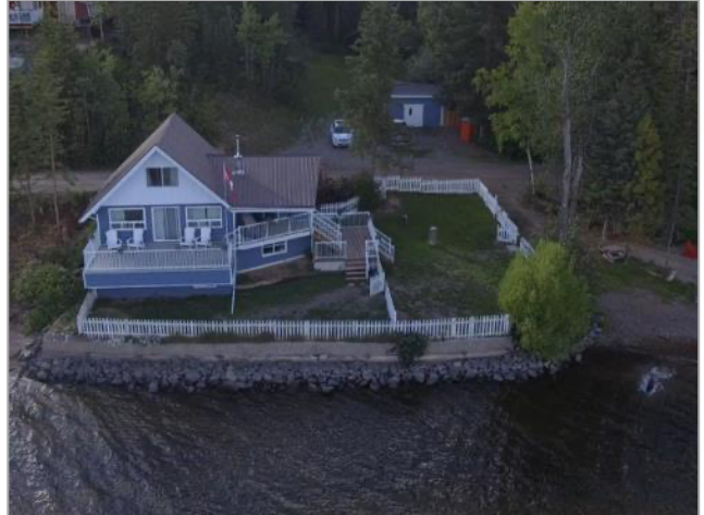
Photo 28. Example of a retaining wall built below the high water mark of the lake (Segment 28).
