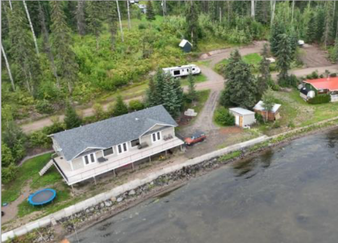
Photo 27. Example of retaining walls built along the shoreline (Segment 29).
