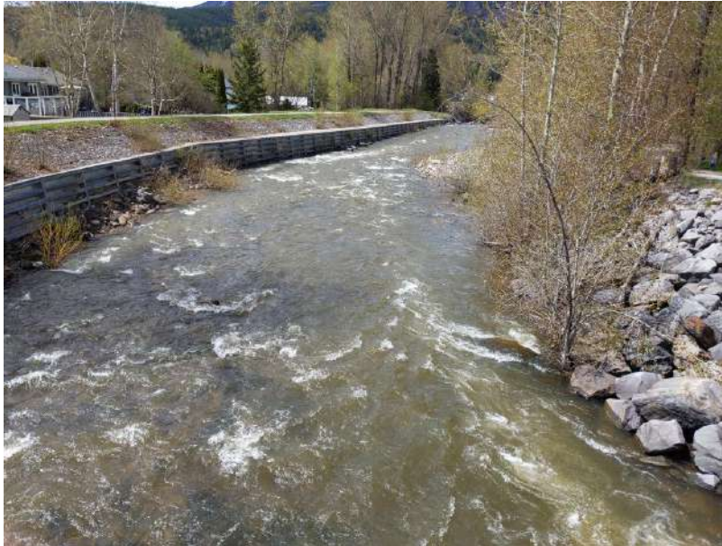
Figure 7: Metal siding (left) clads coal creek. While siding prevents erosion, it provides minimal habitat value or shading. On the right riprap can be seen, this also has minimal habitat value compared to the vegetated riparian zone seen downstream.
