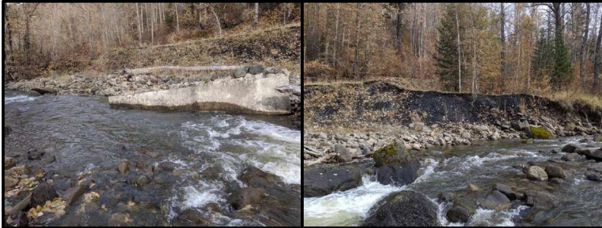
Figure 17. Photos of HACOL01 (Site #17) on Coal Creek.
