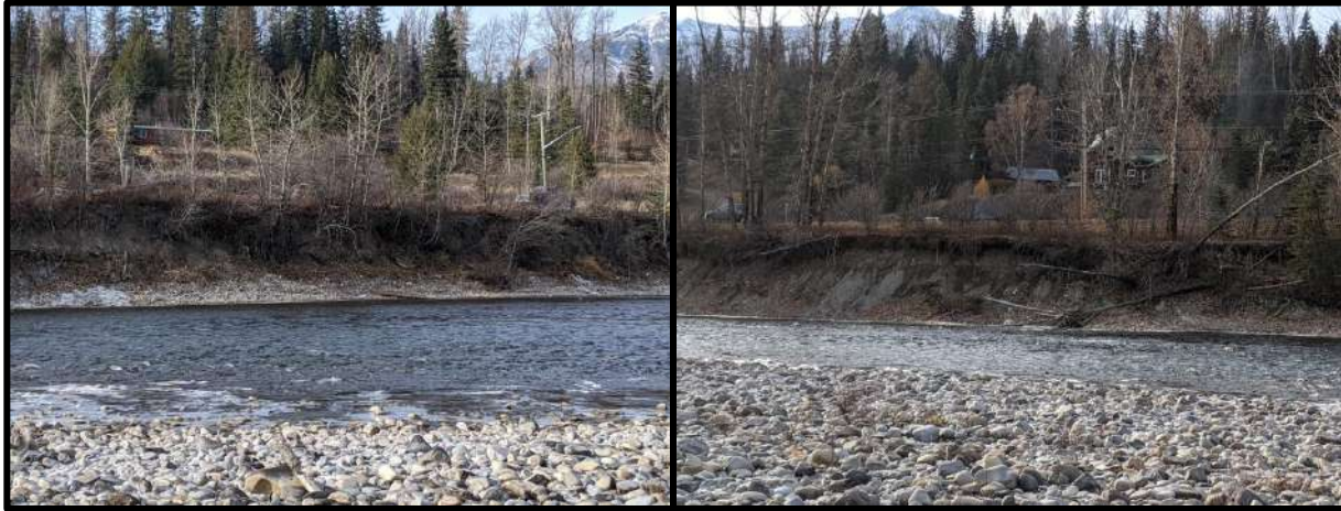
Figure 24. Photos of HAELK03 (Site #7) on the Elk River. These photos illustrate the long section of stream bank that is eroding into the river.
