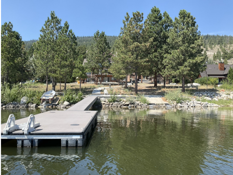
Photo 1: New marina rail, concrete boat launch and dock in Segment 7- Nicola Estates (August 1, 2023).
