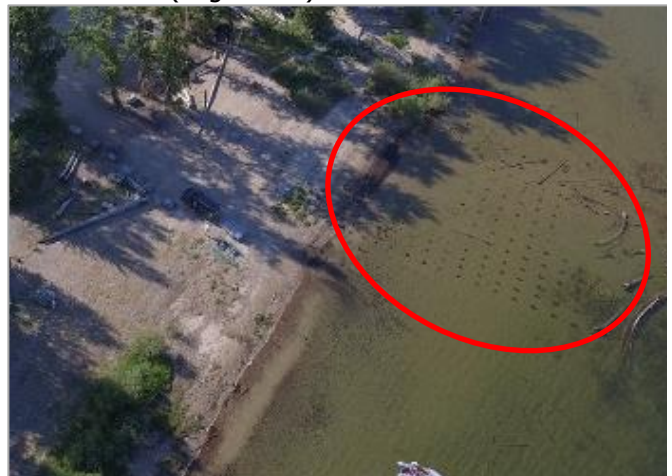
Photo 20. Cut-off pilings near the boat launch (Segment 8).
