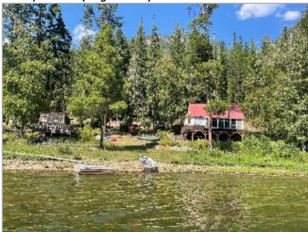
Photo 21. Single family development with dock (Segment 5).
