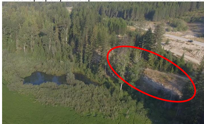
Photo 28. Recent riparian clearing associated with a previously disturbed area at the north end of Segment 3, just south of St. Mary Road.
