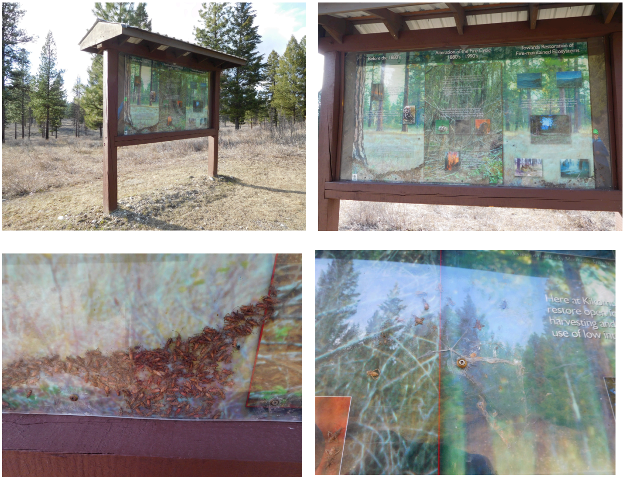
Figure 38: Grassland Restoration Interpretive Kiosk at S030 Top photos are the front of kiosk, bottom photos are of the cracks in the plexi glass and attempted repair, as well as damage due to insects getting in-between the plexi glass and the sign.
