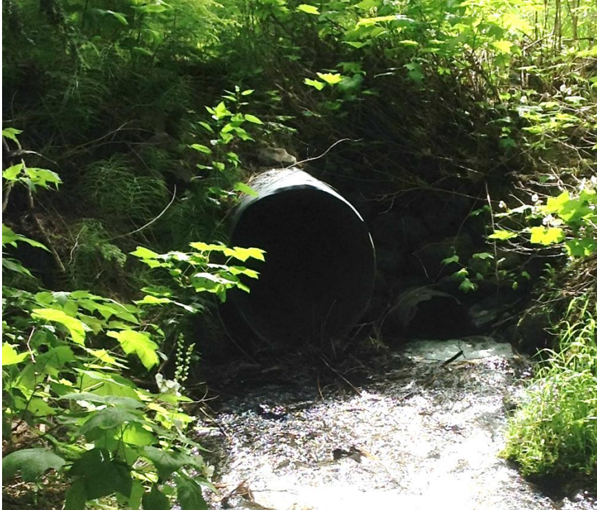
PHOTO 11. BARTLETT CREEK AT STANDARD ROAD. TWO CULVERTS (850MM AND 600MM) APPEAR TO HAVE MANAGED FLOWS ON BARTLETT CREEK WITHOUT INCIDENT FOR AT LEAST SEVERAL DECADES .
