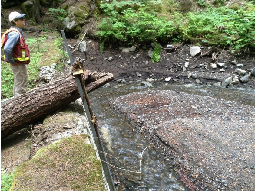
PHOTO 9. THE DAM ON BARTLETT CREEK AT B8. THE LARGER THAN AVERAGE PEAK FLOW IN 2018 HAS DEPOSITED A WEDGE OF SMALL COBBLE TO ORGANIC MUD WHICH IS TRAPPED BEHIND THE DAM.
