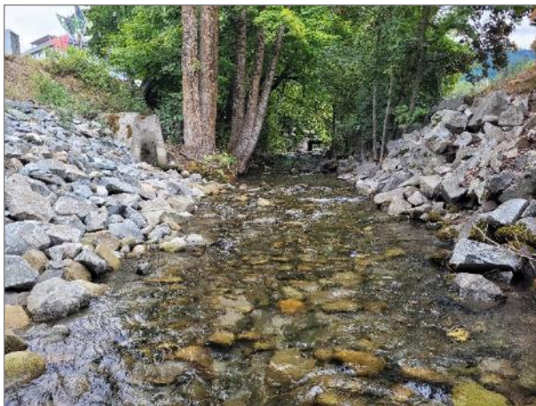
Photo 13. Riprap armoring on both sides of channel, just upstream of Baker Street Bridge.
