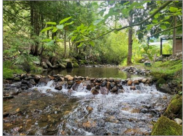
Photo 30. Constructed dam next to a residential property forming a fish barrier during low flow conditions.
