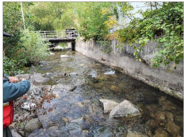
Photo 14. Concrete wall on east bank of the creek within R2-S2.
