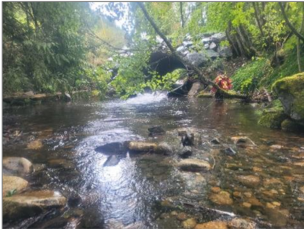
Photo 46. Proposed location for weir leading up to Kline Road culvert.
