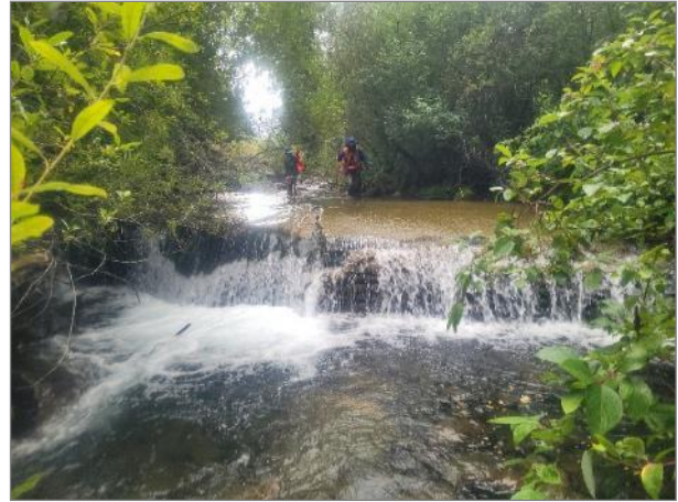
Photo 20. Small falls created by a constructed dam/platform at the upstream end of Site 5.
