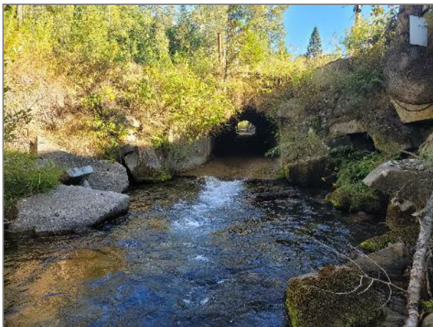
Photo 48. Proposed location for weir leading up to Highway 6 culvert.
