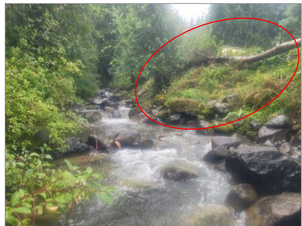
Photo 22. Riparian vegetation removal and relic riprap armoring on the east bank of R3-S2.
