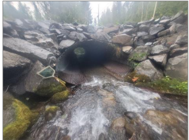
Photo 47. Kline Road culvert outlet.
