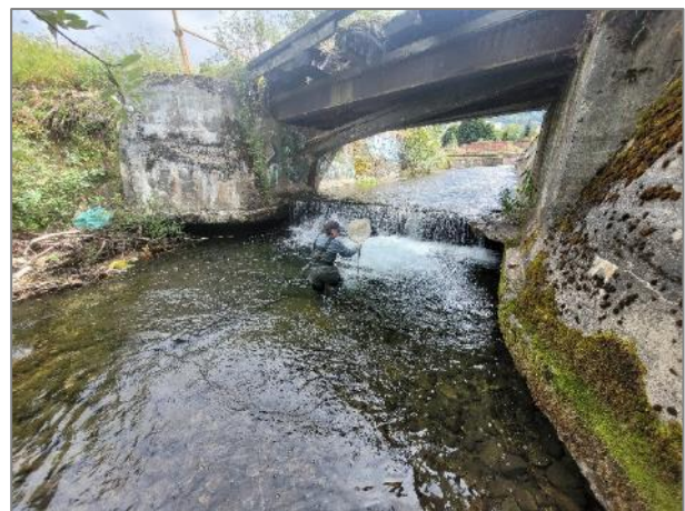
Photo 44. Drop at flume outlet.
