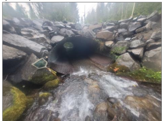
Photo 28. Upstream view of culvert outlet under Kline Road.
