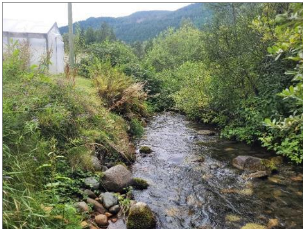
Photo 25. Residential property with channel armoring on east bank of Cottonwood Creek (facing upstream).
