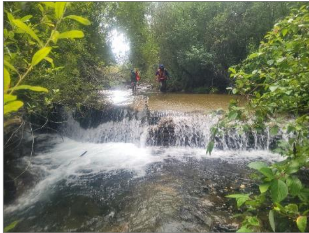
Photo 45. Constructed dam/platform proposed to be replaced with a weir.
